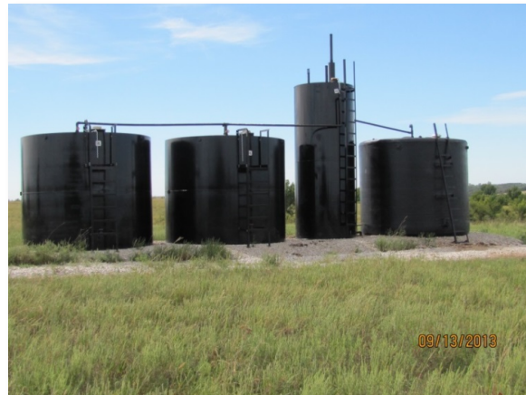
George Prospect Tank Battery
