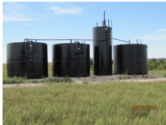
George Prospect Tank Battery
