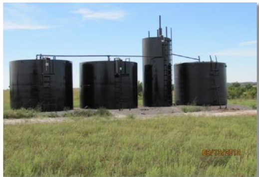
George Prospect Tank Battery
